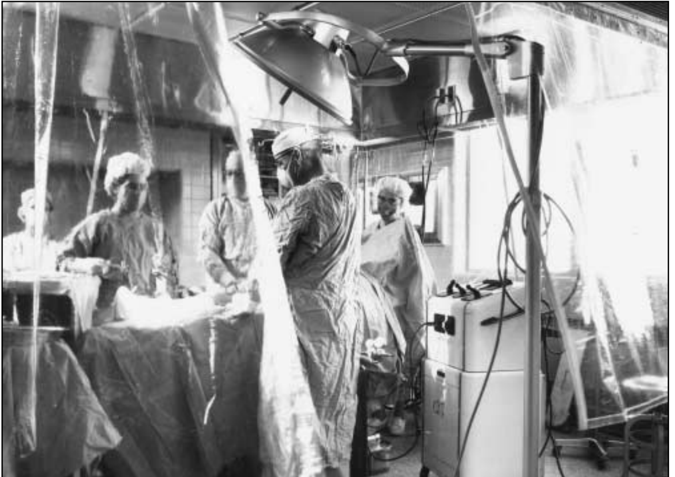
Vertical Flow Curtain Room (Portable) This is the first laminar flow operating facility in the world. It had plastic curtains at the side and used vertical laminar flow from HEPA filters suspended from the ceiling above the operating table. Six blowers provided vertical air flow of 90 feet per minute or about 600 air changes an hour. Details of its design, construction and testing can be found in Reference 5.
